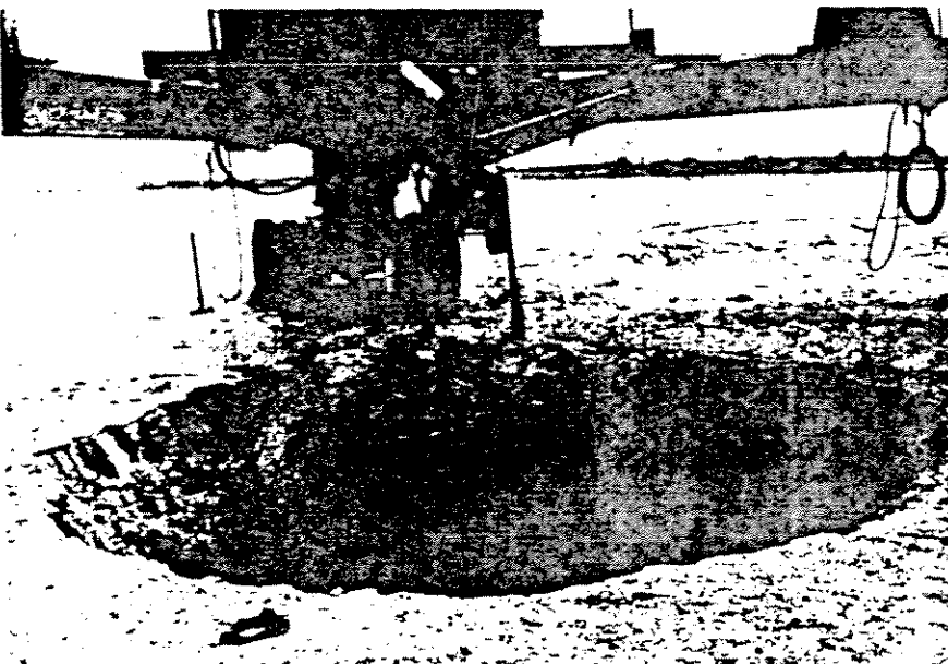
Photo B Crater formations made after pounding process is completed.
