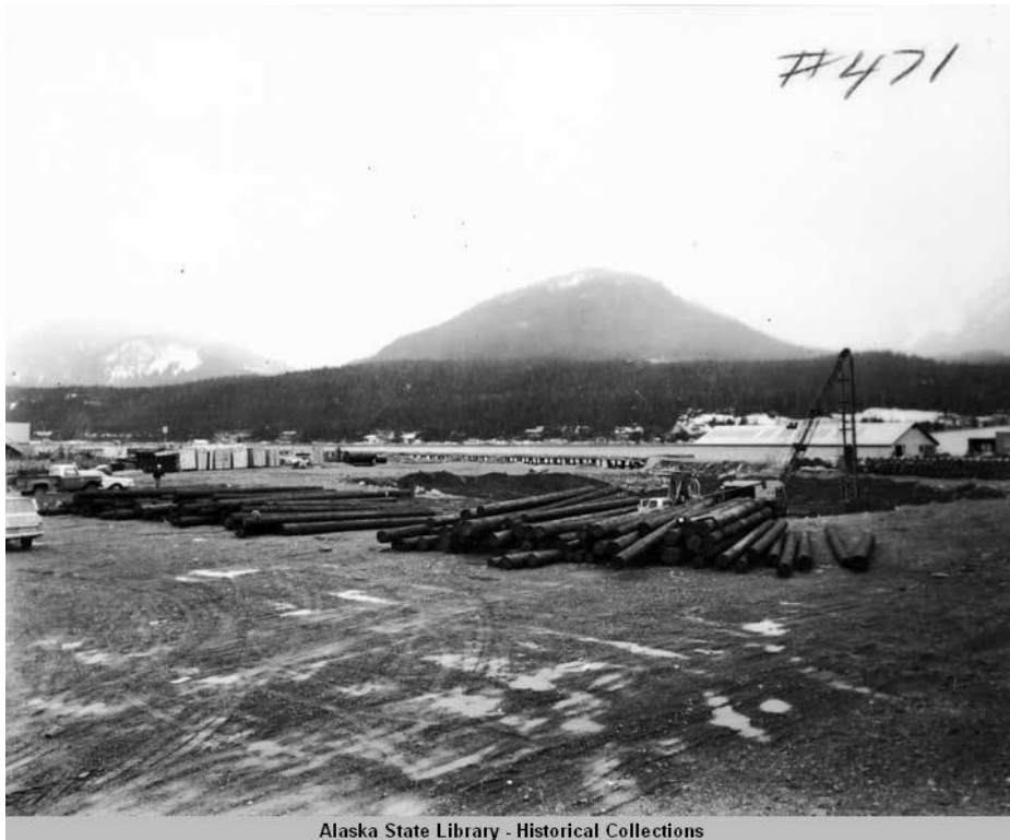
Figure-1. Photo showing the timber logs that was likely used as piles.
