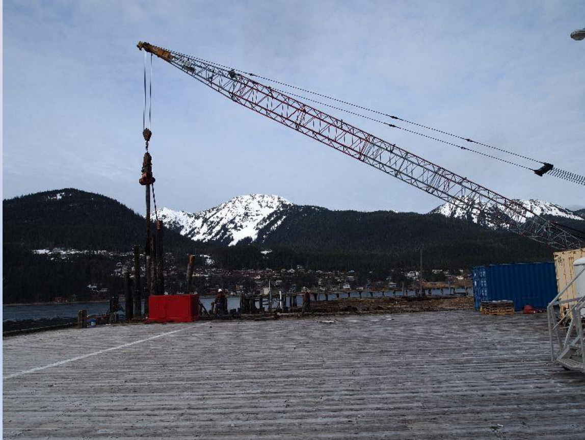
The crane lifts a piling.
