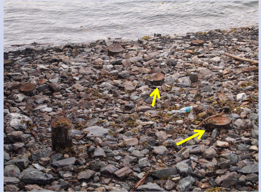
Views of the beach that is under the old dock. Pilings closer to the shore are cut off as opposed to being removed.
