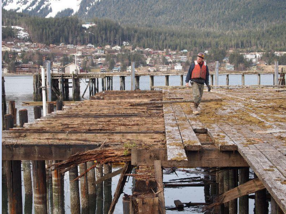
The deck during the demolition process.
