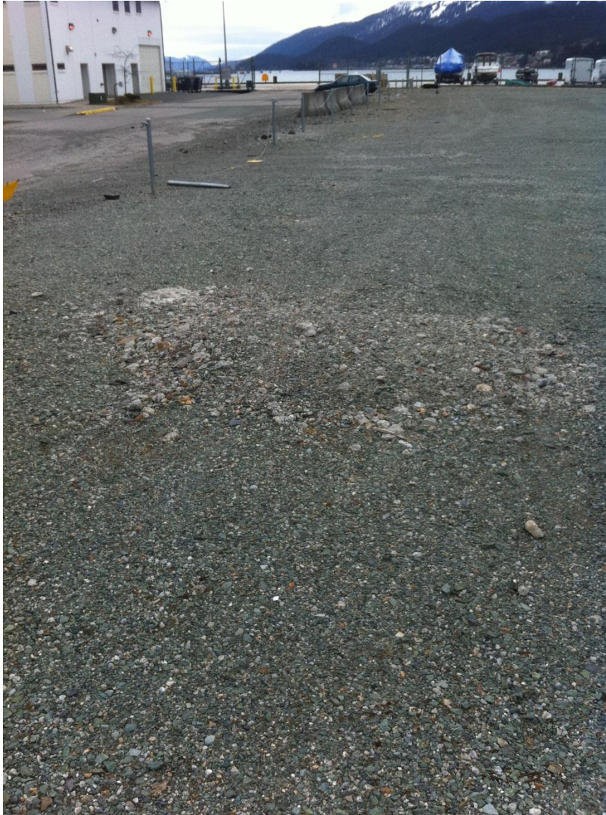
Photograph 8. Mounded area of gravel located to the north of the Whittier Street vehicle access.
